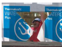
On arrival of doors and windows, cut Watergate at each opening on a 45° angle away from each corner. Pull the Watergate flaps inside and fasten to the inside of frame.
